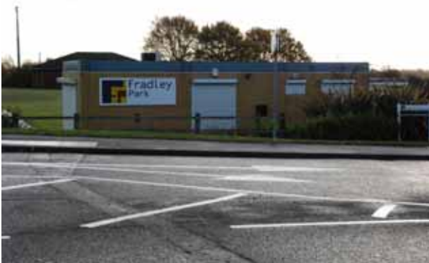
The Parish Council office, Wellington Crescent, Fradley Park
