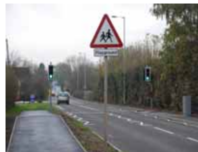
Streethay Pedestrian Crossing
